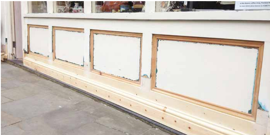
Figure 56. Timber stallriser repair
