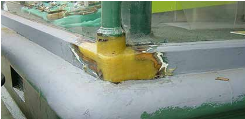
Figure 55. Resin repair to timber shopfront detail
