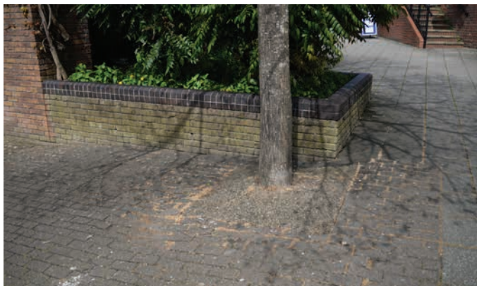
Existing tree roots damaging paving area
